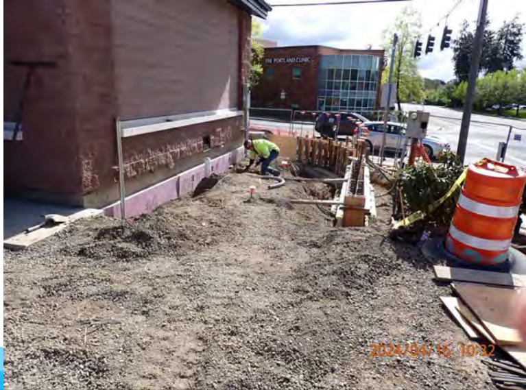
Sitework at exterior of PFC Facility
