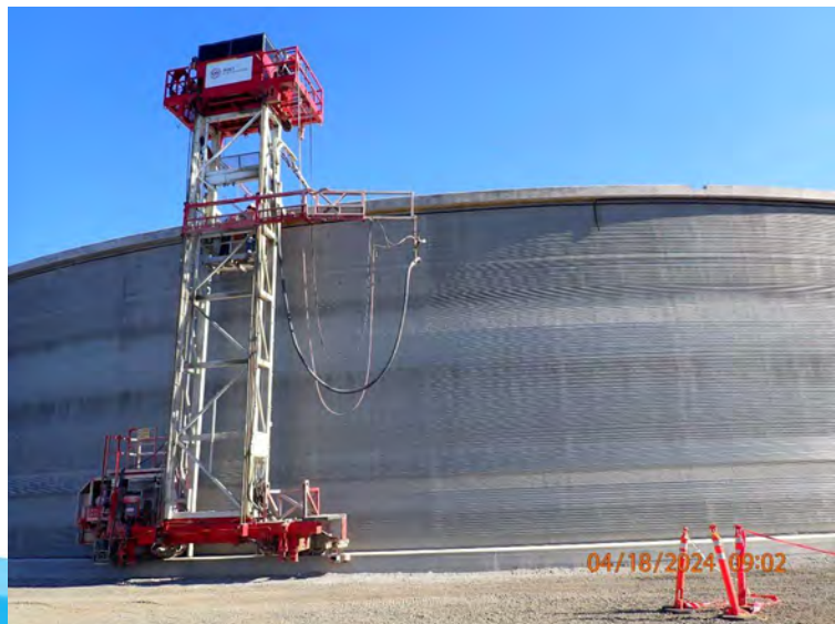
Preparing for final shotcrete application to tank
