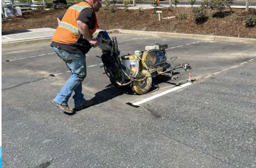
Striping parking lot at Reedville Creek Park
