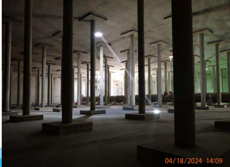
Interior of reservoir tank
