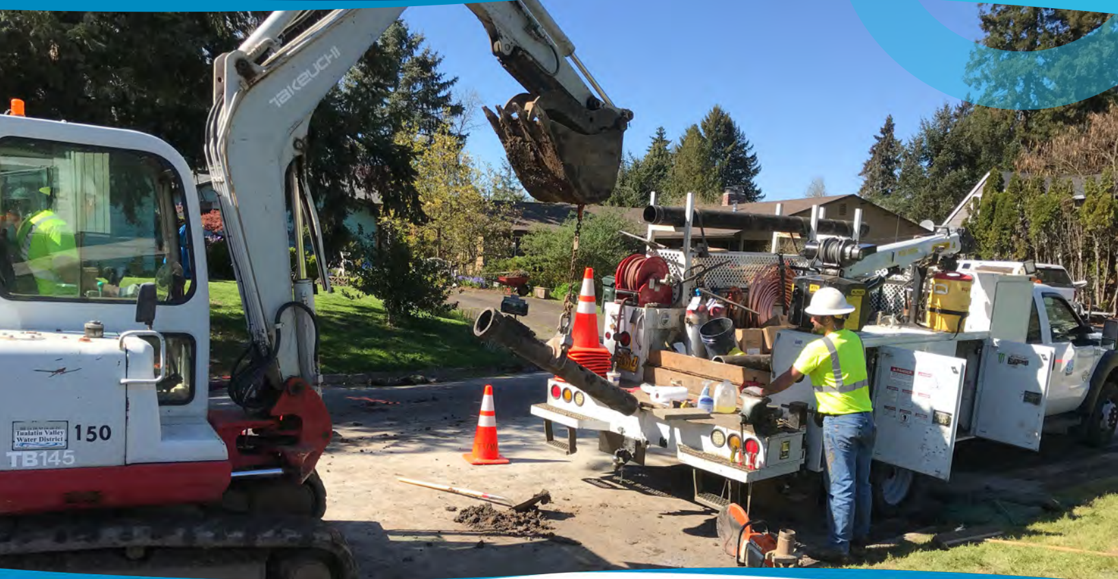
Crews replace a water main
