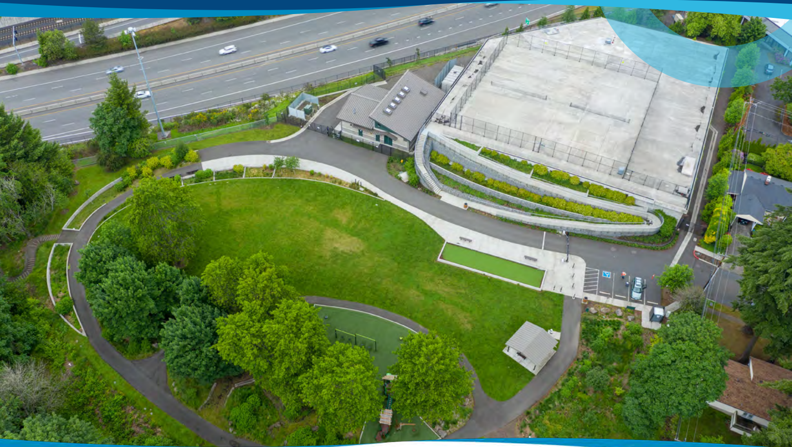
Ridgewood View Reservoir and Pump Station
