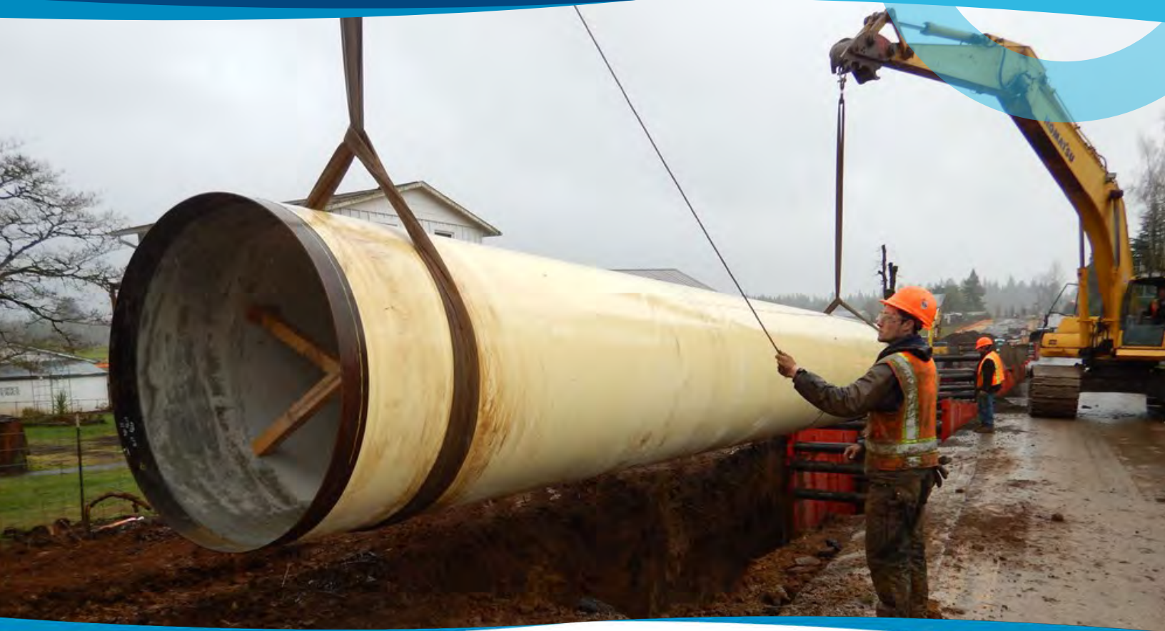
Pipe installation for the Willamette Water Supply System
