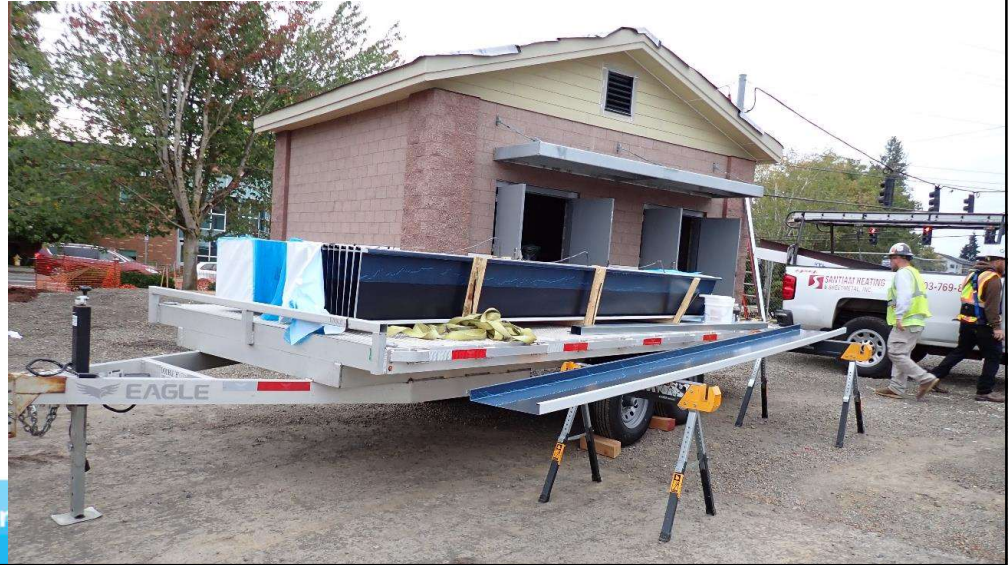
PFC Building roof installation
