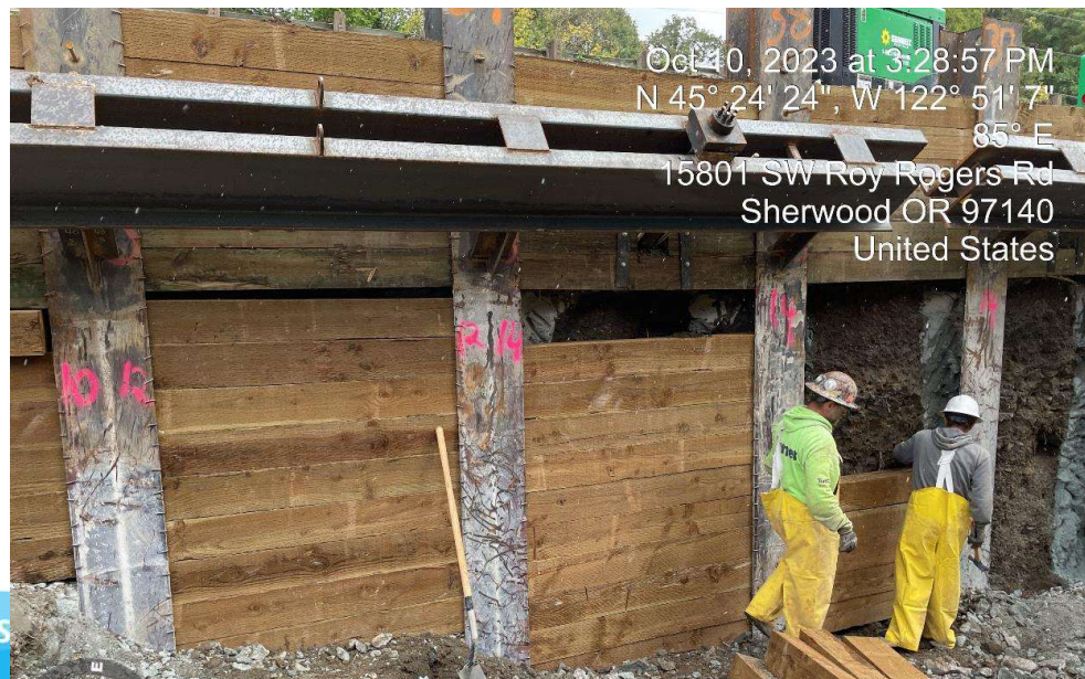
Installation of retaining wall at Tributary #4
