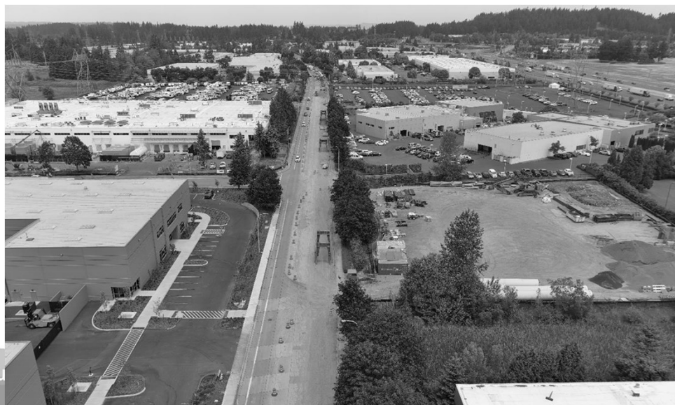
Waterline installation on 95 th Avenue
