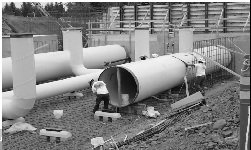
Area 28 & 30 Under slab Piping
