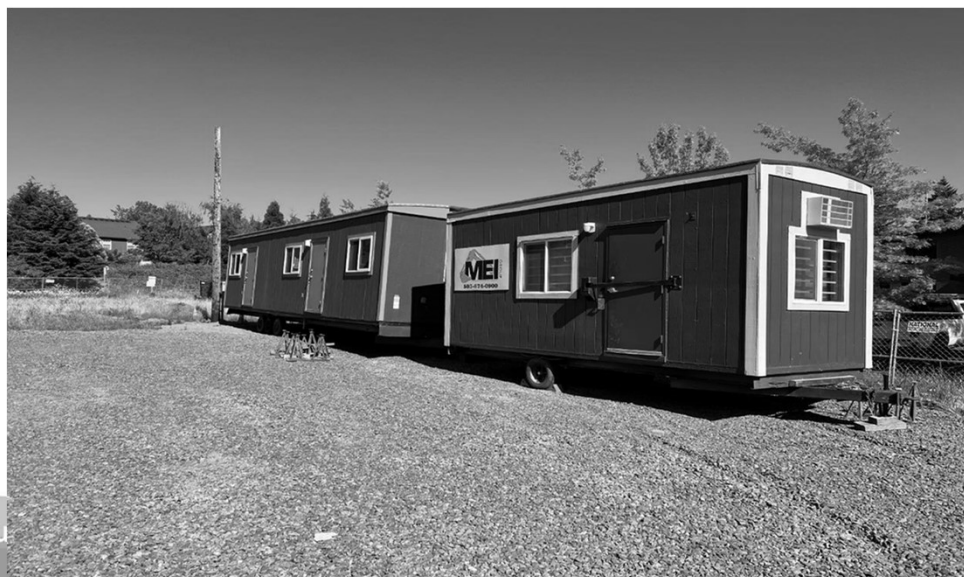
Construction trailers arrive at staging area
