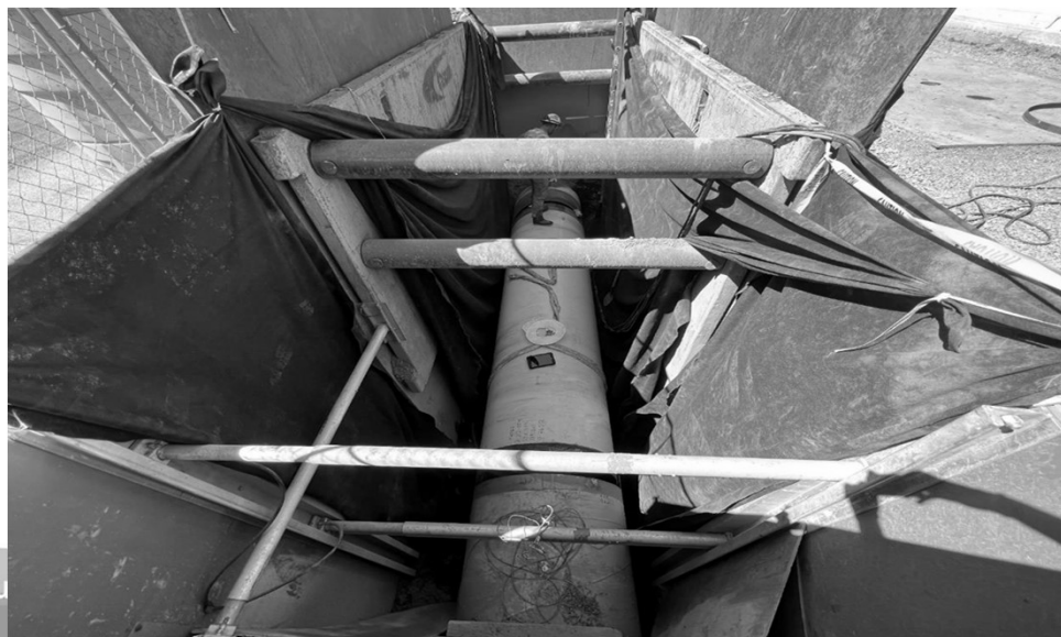
Connection of 48" waterline to PLW_1.1
