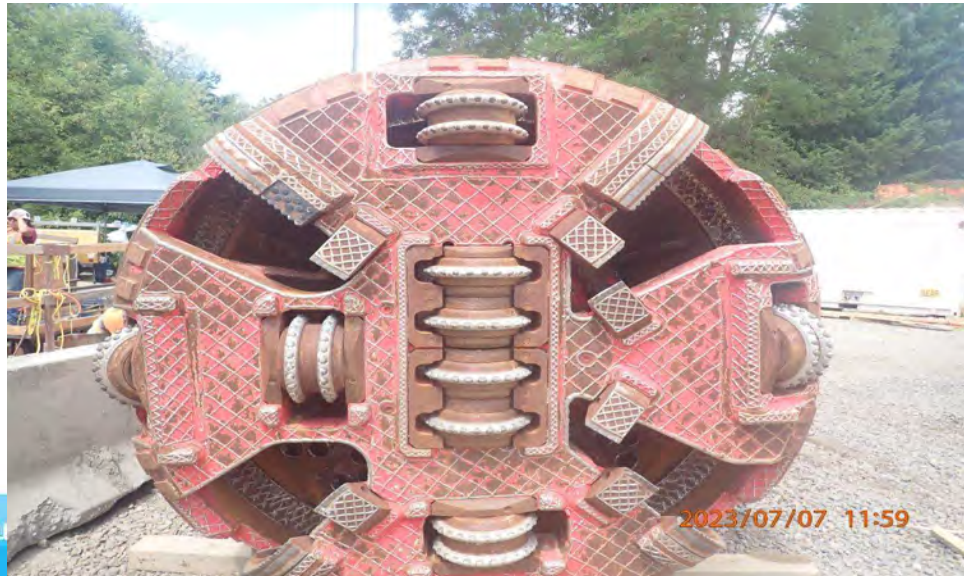
Chicken Creek Crossing MTBM arriving on site
