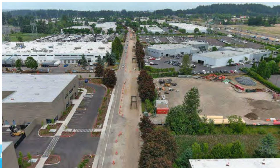
Waterline installation on 95 th Avenue
