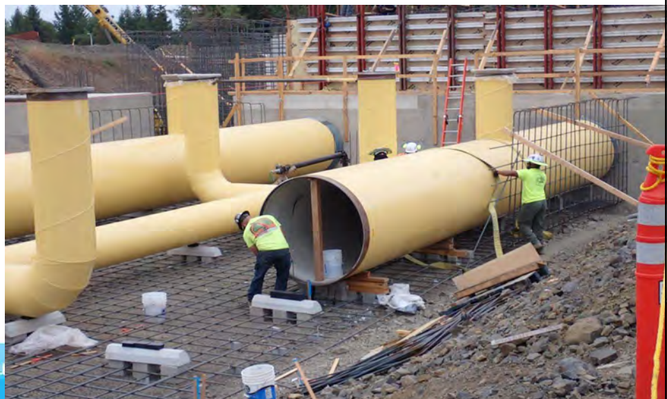
Area 28 & 30 Under slab Piping
