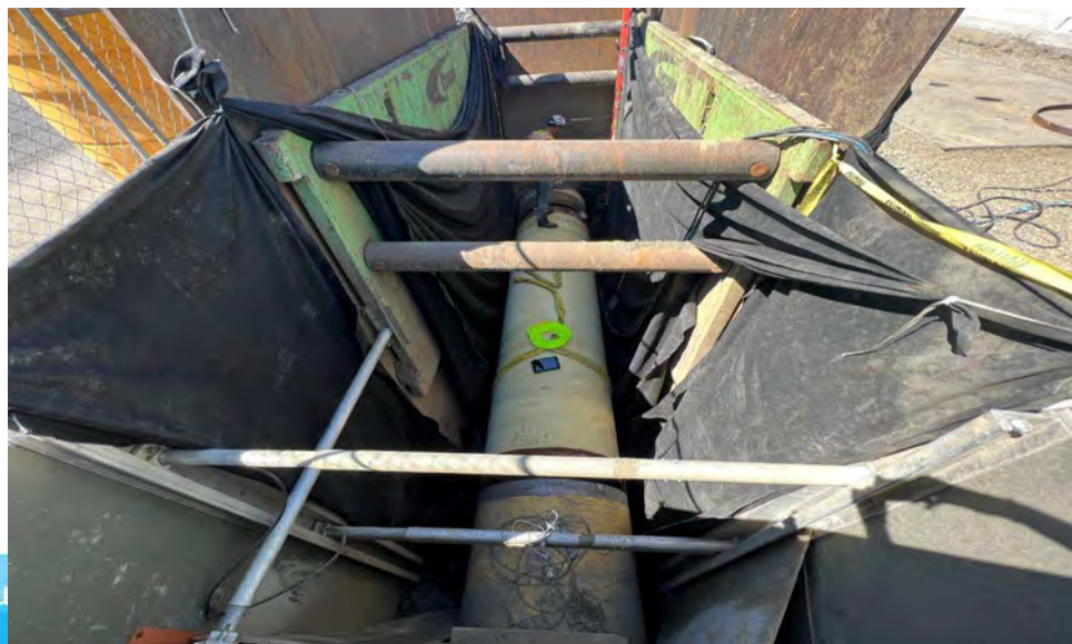
Connection of 48" waterline to PLW_1.1
