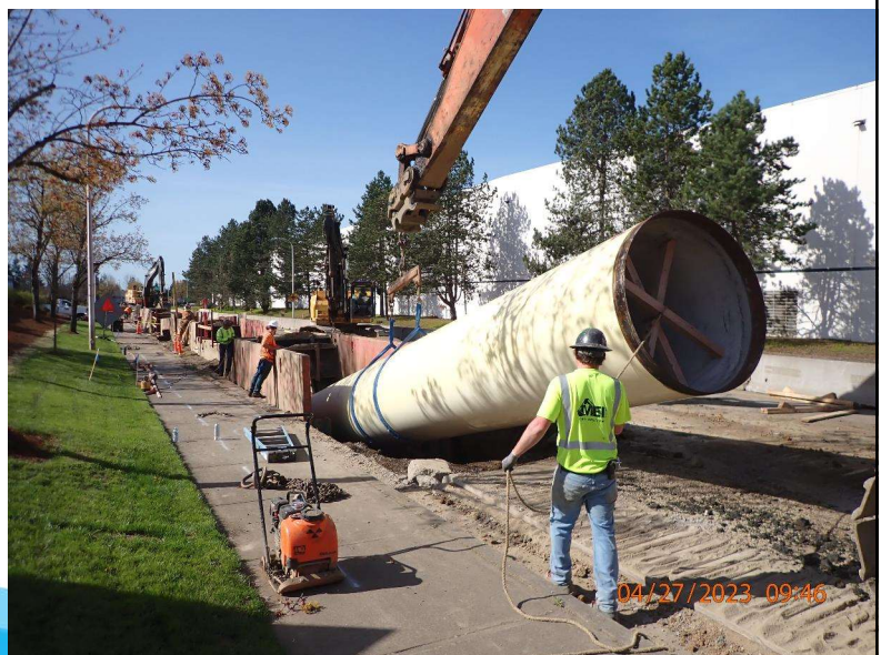
66-inch pipe installation on 95 th Avenue
