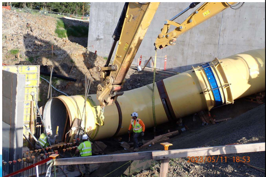
84-inch yard pipe at FWPS
