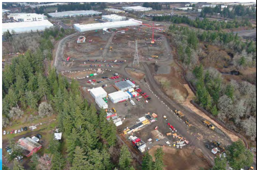
WTP site looking northwest
