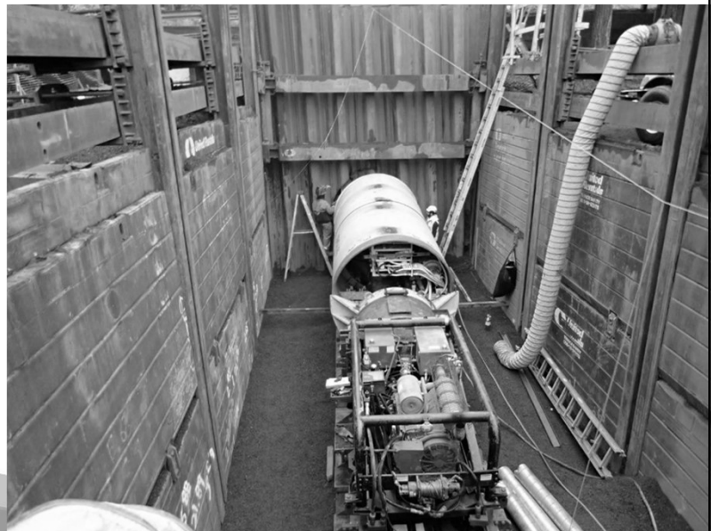
Trenchless crossing under Farmington Road
