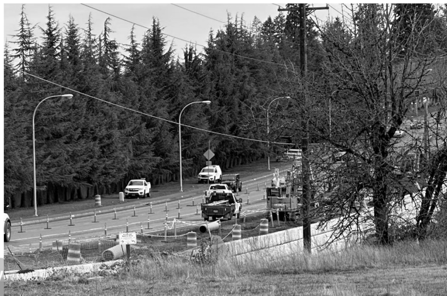
Retaining wall work along Tualatin-Sherwood Road
