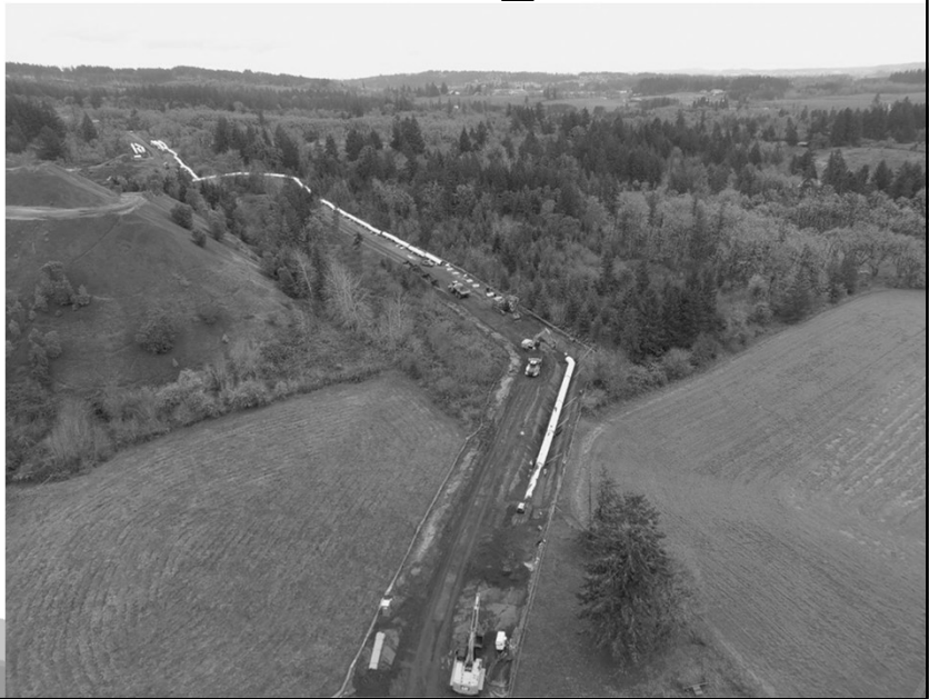
Installing the 66" pipeline
