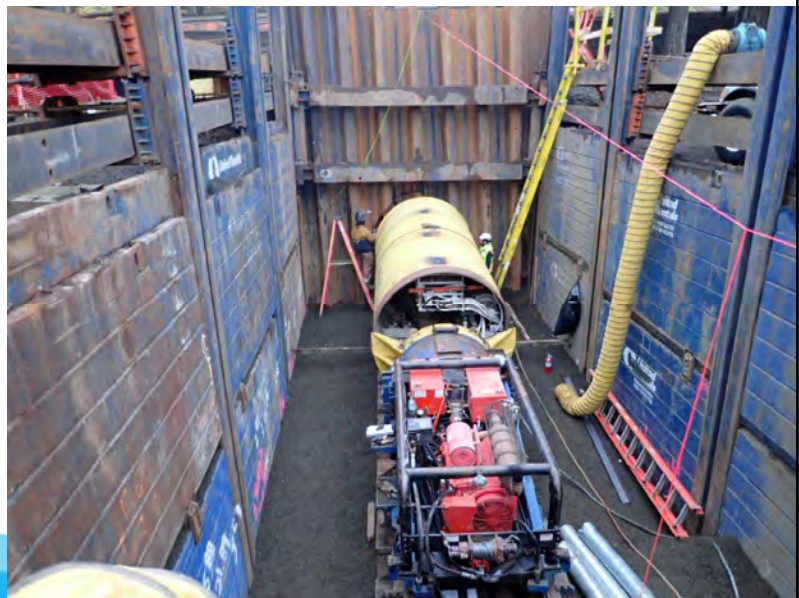
Trenchless crossing under Farmington Road
