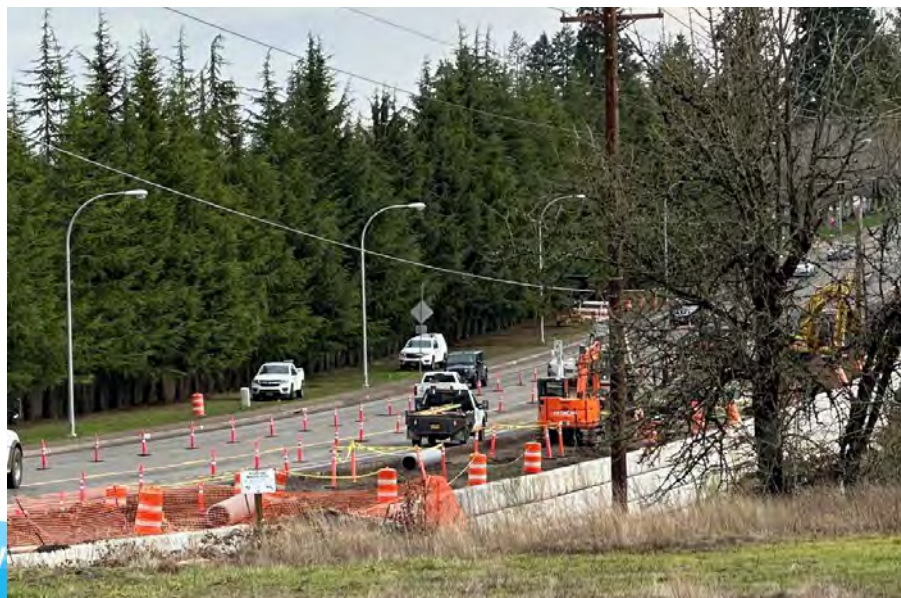
Retaining wall work along Tualatin-Sherwood Road
