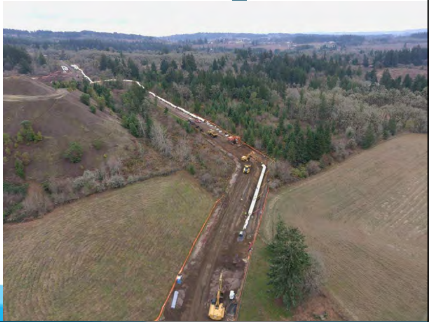
Installing the 66" pipeline
