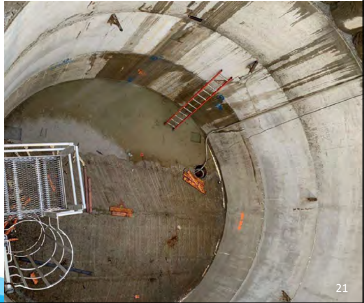
South shaft setup for microtunnel boring machine
