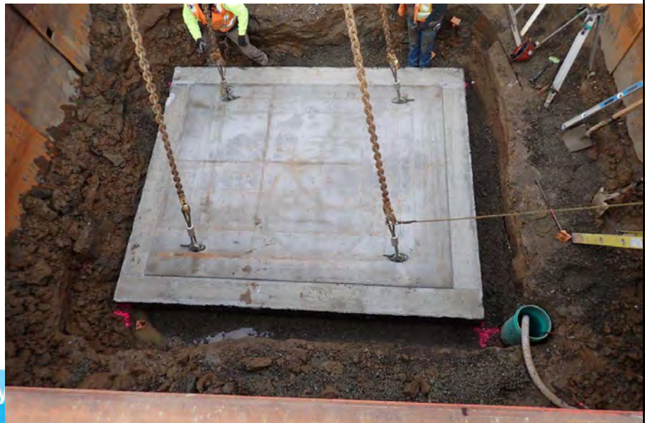
PFC flow meter vault base
