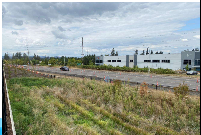
Road work along Tualatin-Sherwood Road
