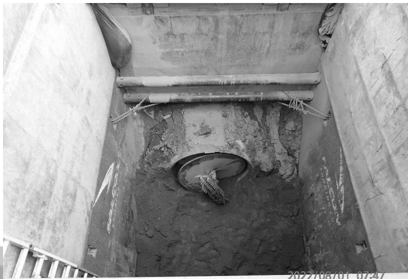
Auger bore tunnelling machine breaking into receiving shaft
