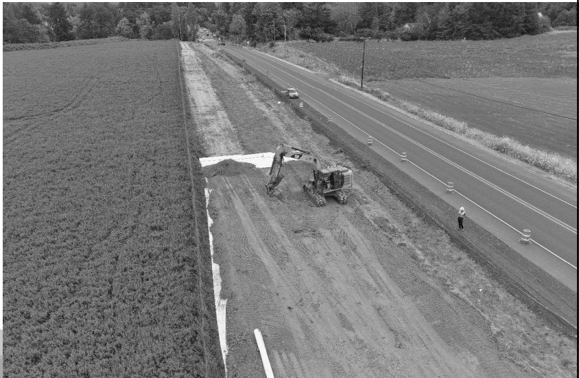
Access/haul road construction for waterline alignment
