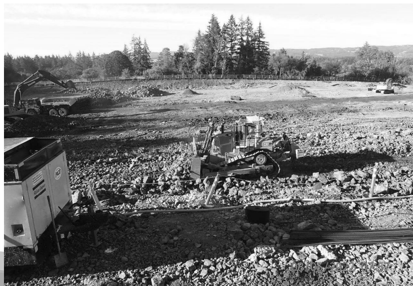
Excavation at RES_1.0 site
