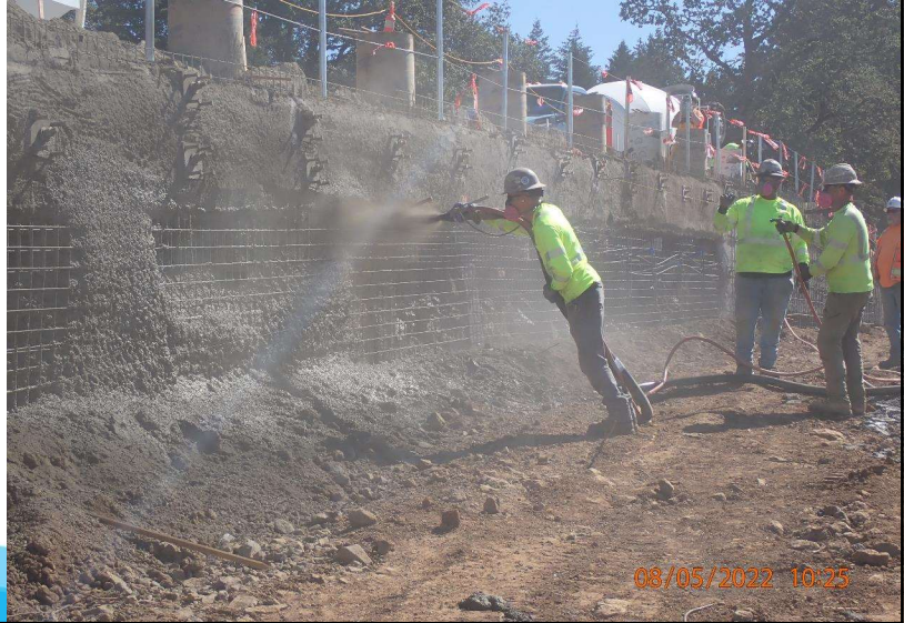
Shotcrete placement for soil nail wall at RES_1.0 site
