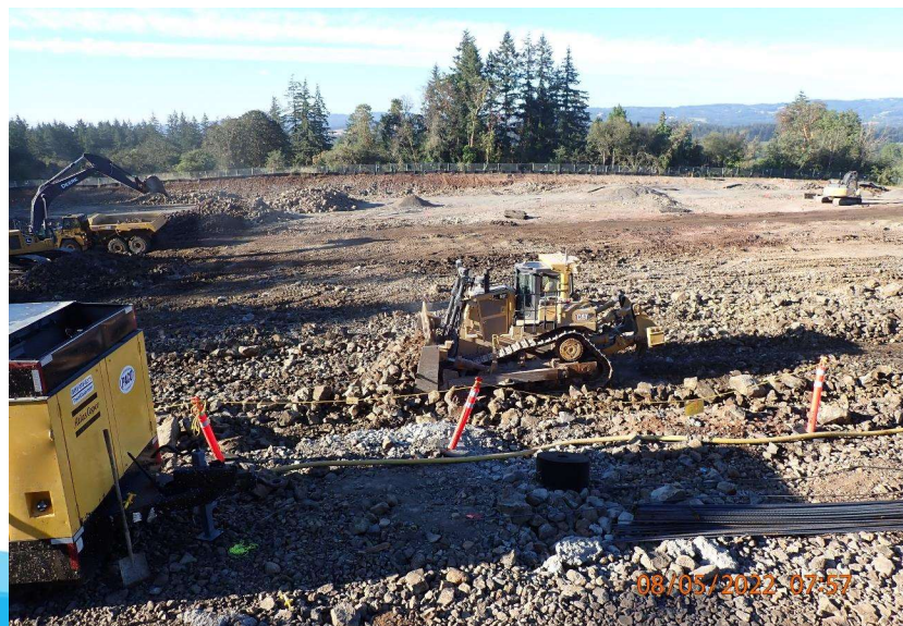
Excavation at RES_1.0 site
