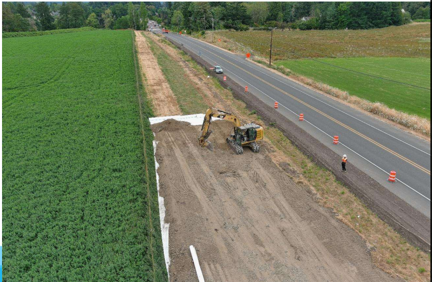
Access/haul road construction for waterline alignment
