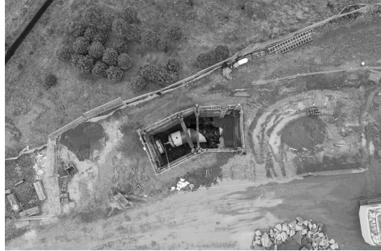
Connection to adjacent PLM_1.1 pipeline
