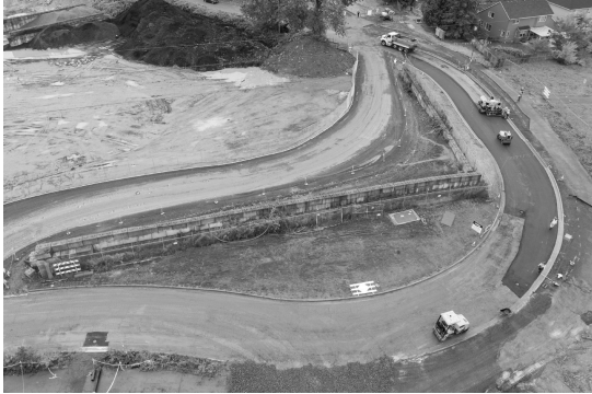
Pinch point pavement replacement
