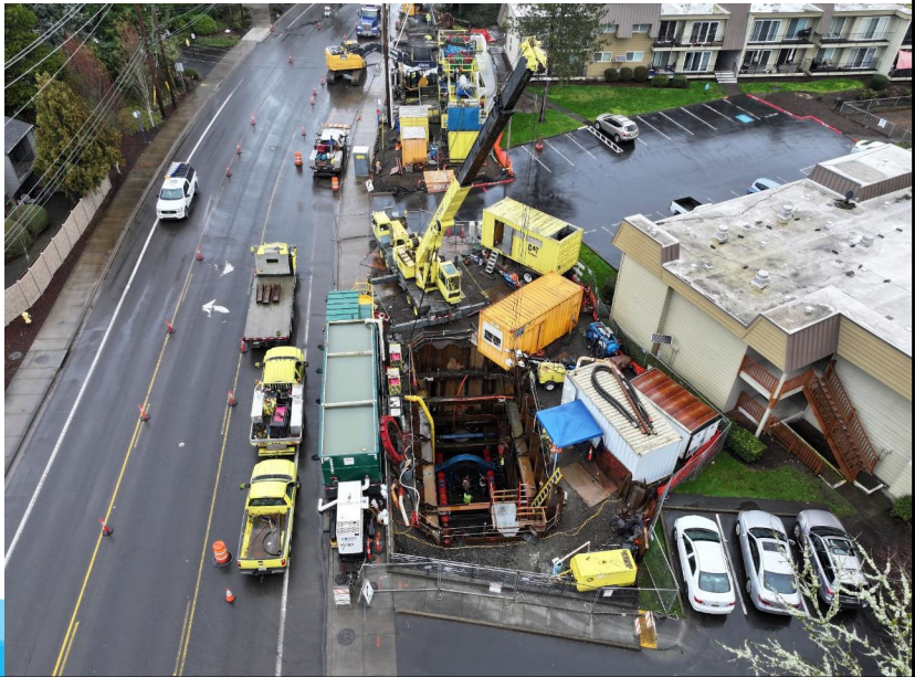
Upper Fanno Creek trenchless crossing site
