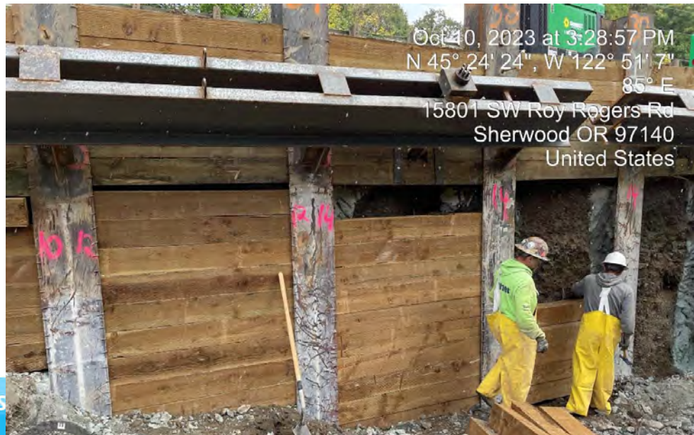
Installation of retaining wall at Tributary #4
