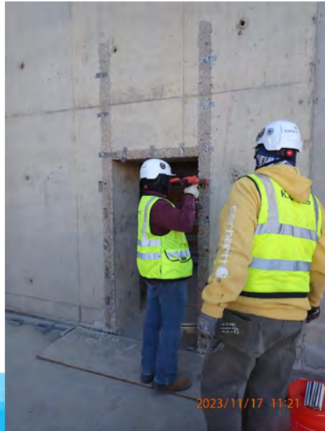
Slide gate installation at EQ Basin
