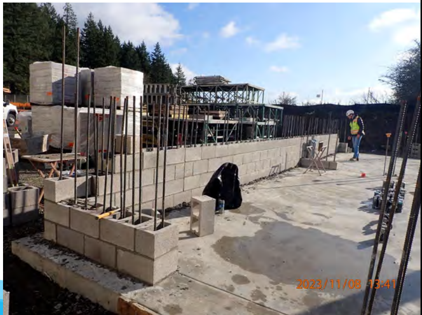
Water Quality Building masonry walls
