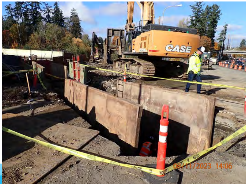
48-inch waterline installation in Cornelius Pass Rd. near entrance to Orenco Woods Nature Park
