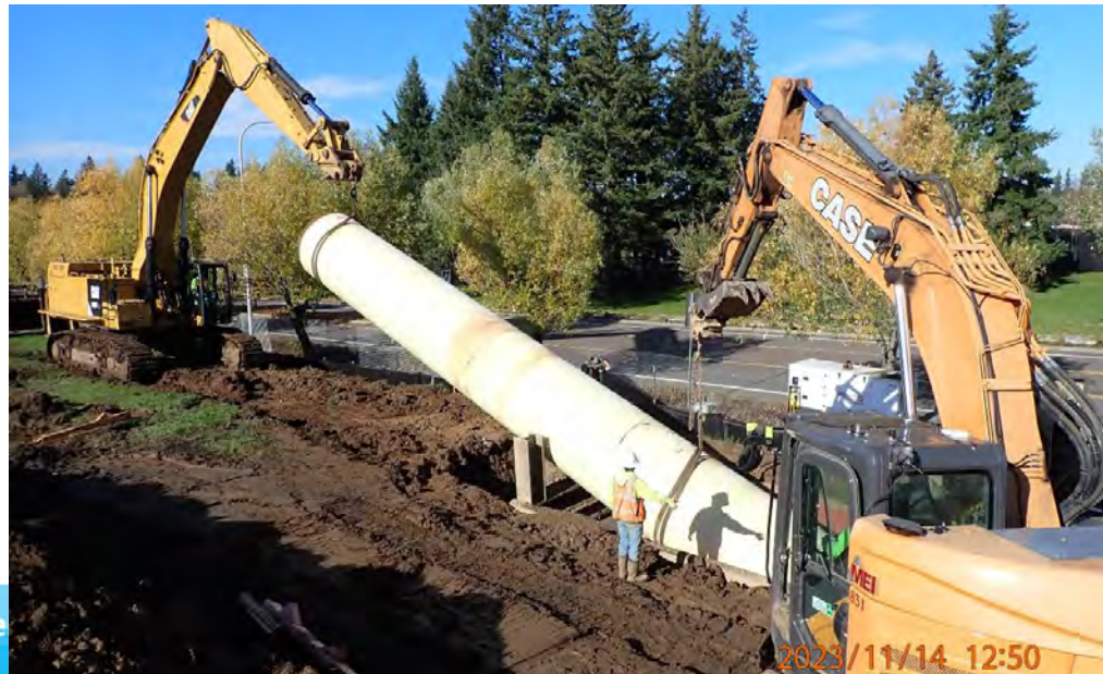
66-inch waterline installation near Boeckman Rd.
