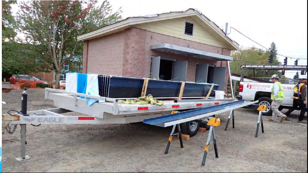
PFC Building roof installation
