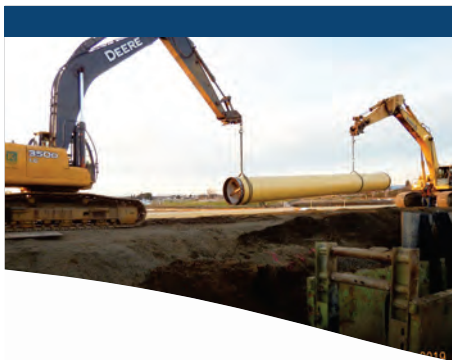
Construction of the additional water supply
