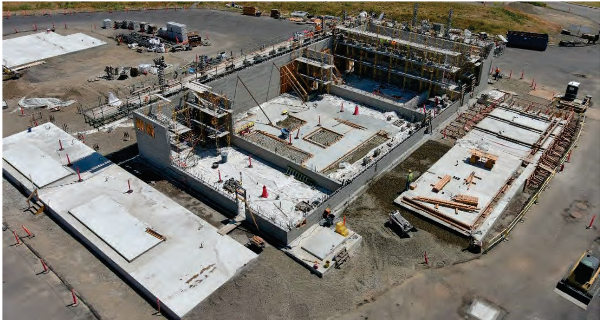
Upper Site: Electrical Building CMU wall progress. Backfilling around Transformer slab.
