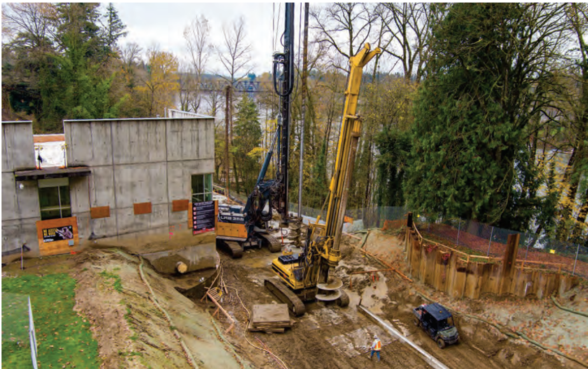
Seismic improvements at the river intake
