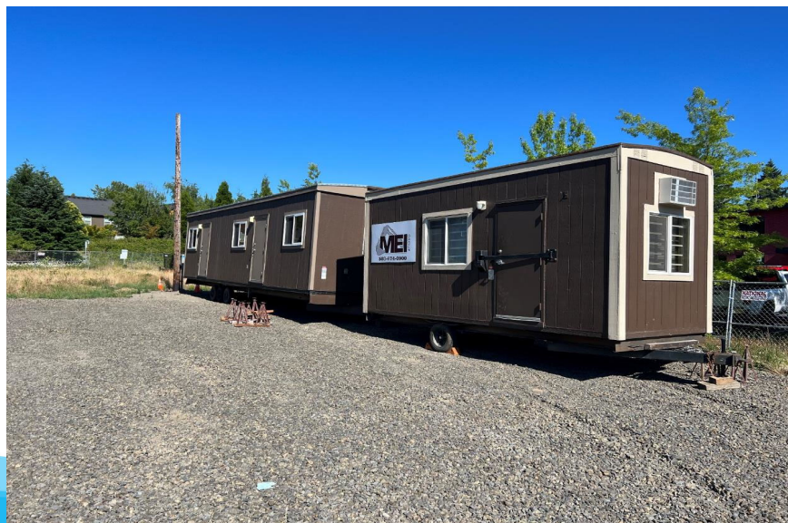
Construction trailers arrive at staging area
