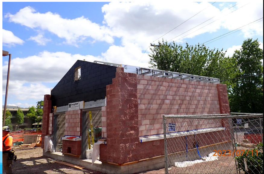
PFC Building CMU walls and steel trusses
