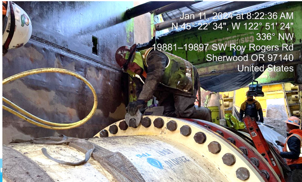
66-inch butterfly valve installation
