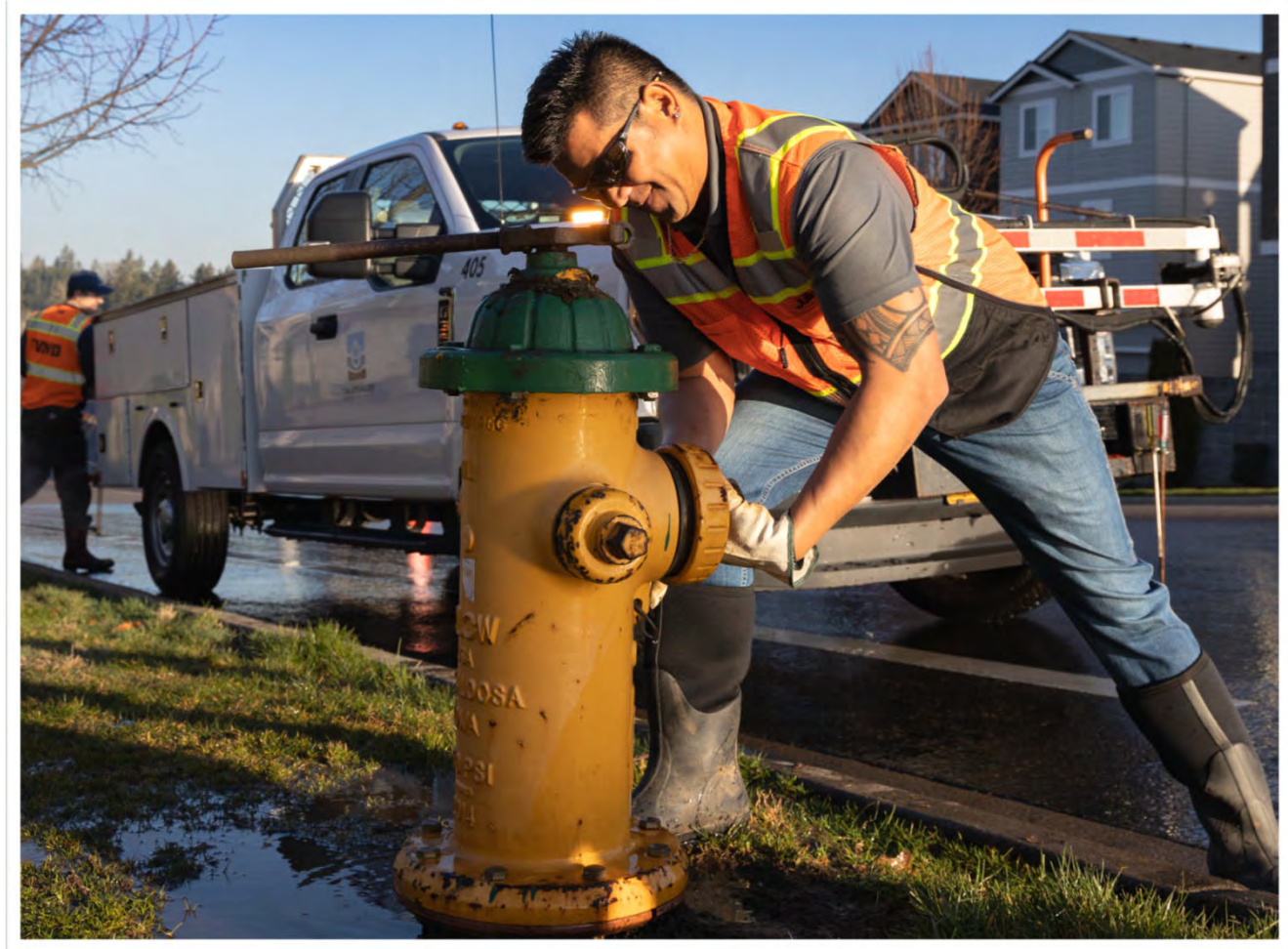
TVWD Operators performing maintenance on a hydrant
