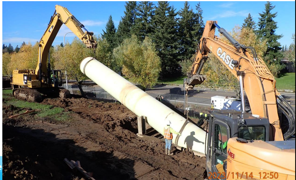
66-inch waterline installation near Boeckman Rd.
