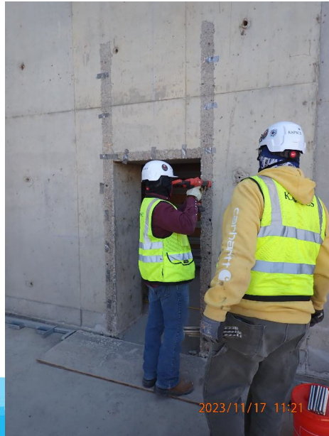
Slide gate installation at EQ Basin
