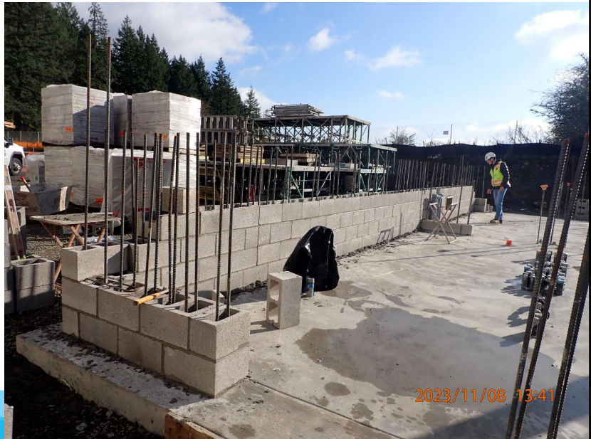
Water Quality Building masonry walls
