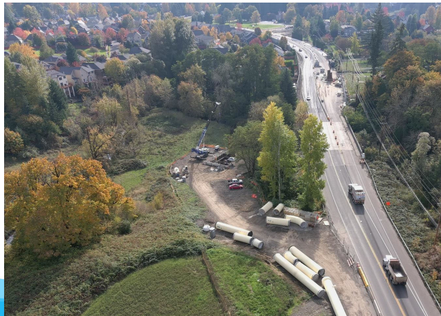
Chicken Creek tunnel shaft shoring removal
