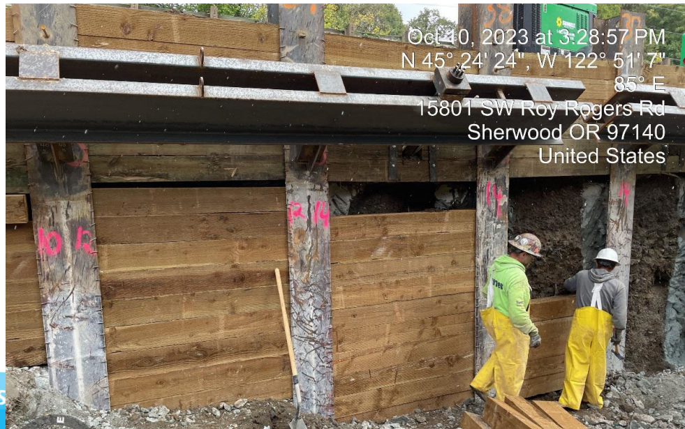
Installation of retaining wall at Tributary #4
