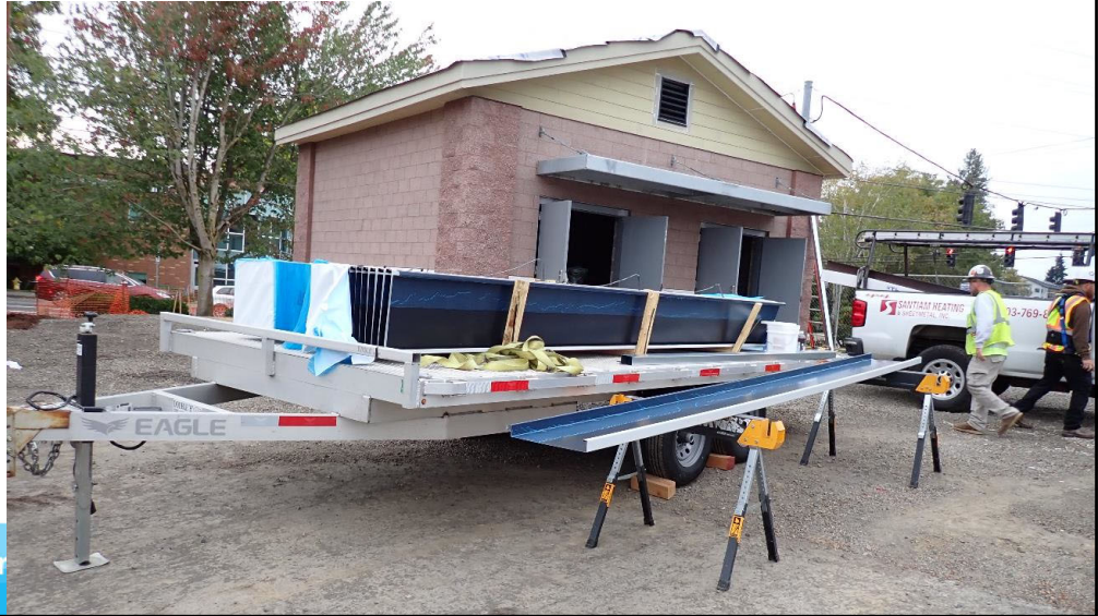
PFC Building roof installation
