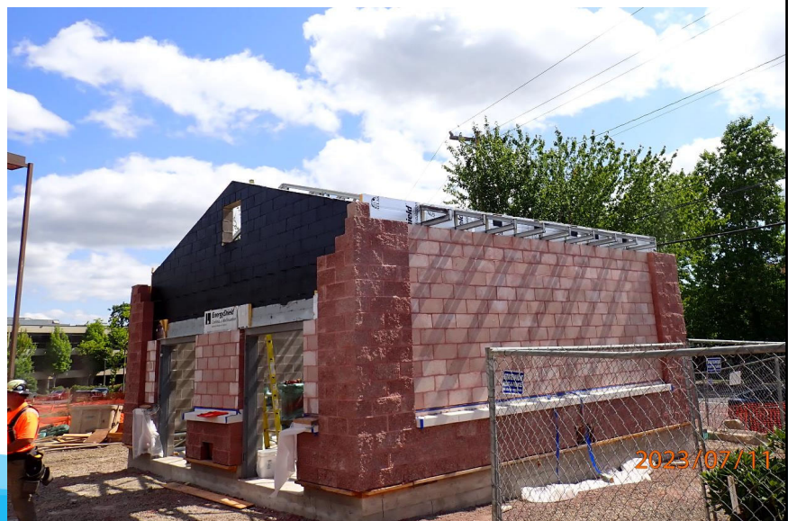
PFC Building CMU walls and steel trusses
