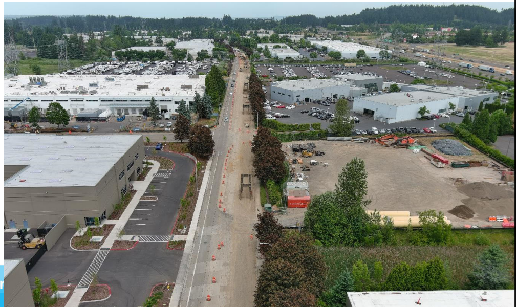
Waterline installation on 95 th Avenue
