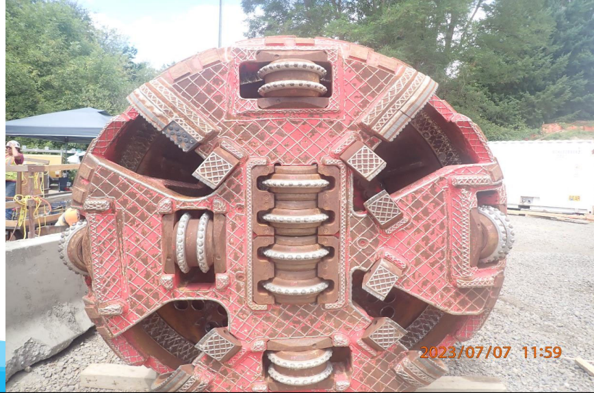
Chicken Creek Crossing MTBM arriving on site
