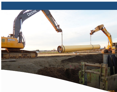
Construction of the additional water supply
