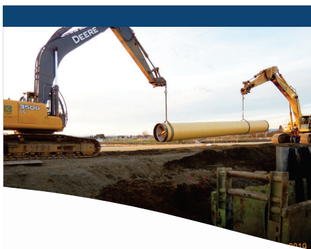
Construction of the additional water supply
