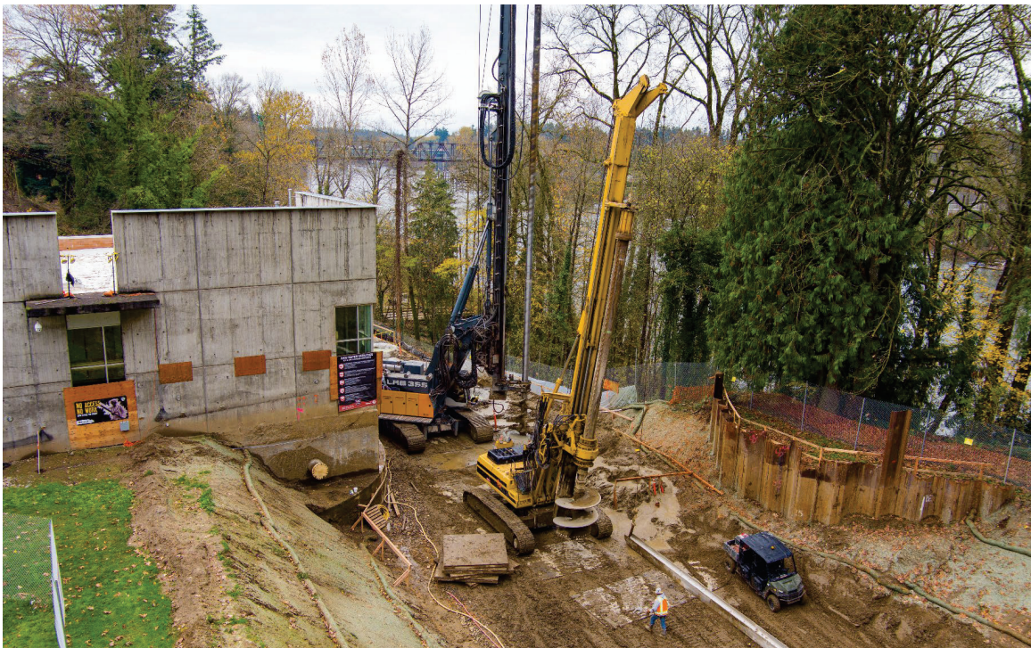
Seismic improvements at the river intake
