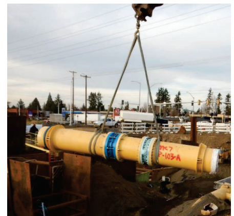
South Hillsboro Area Pipeline Project Coordinated with Newland
